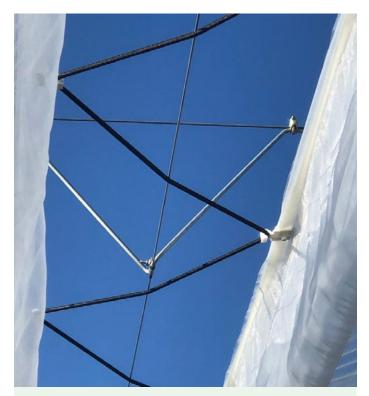
Extremely high wind stability due to an efficient combination of bungy systems, eaves wire and transverse bracing (solid upwards and elastic downwards).
